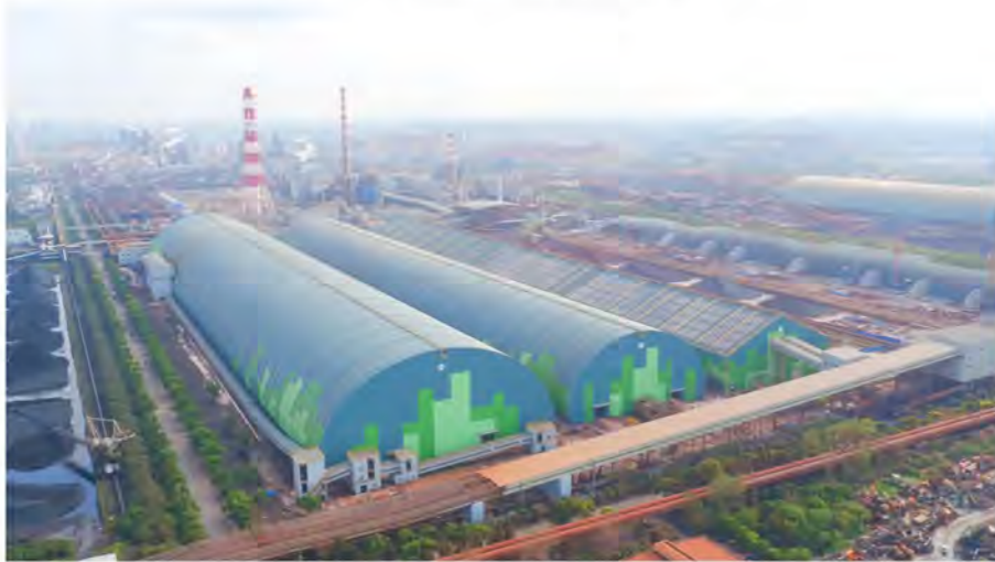
Baosteel's Ironmaking Plant has become greener thanks to its new eco-friendly stockyard
