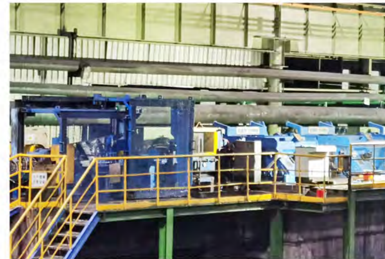
The finishing mill rebuild area of the high-speed wire-rod rolling line
