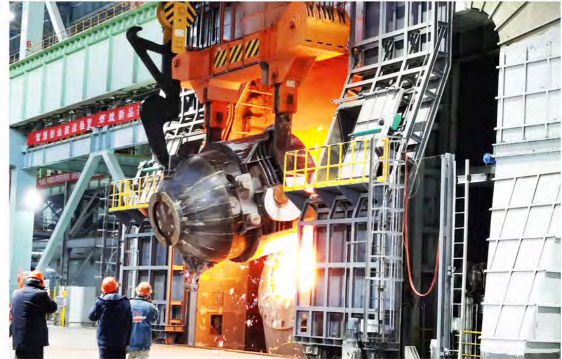
The two BOFs, both built by CISDI, are operating in sync at Shandong Steel's Laiwu Plant
