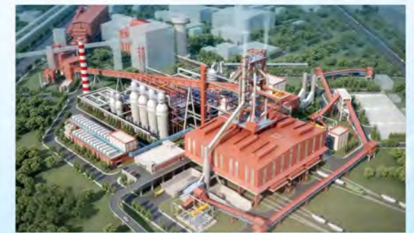
Design and core equipment supply for blast furnace 2 at TATA Steel Kalinganagar Plant, the world's largest new blast furnace under construction (volume 5,870m 3 )
