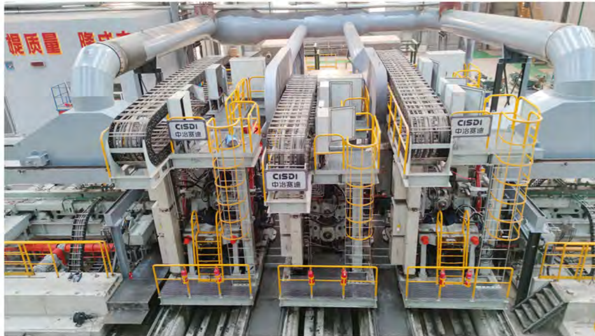
The CISDI-supplied UMCD Universal Mill, installed at Yongyang Special Steel
