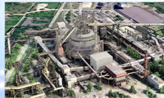
Design and core equipment supply for a 5,050m 3 blast furnace rebuild at ArcelorMittal's Ukraine plant
