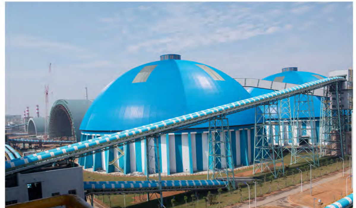
CISDI-built green, smart stockyard at Baosteel Zhanjiang in China's Guangdong Province
