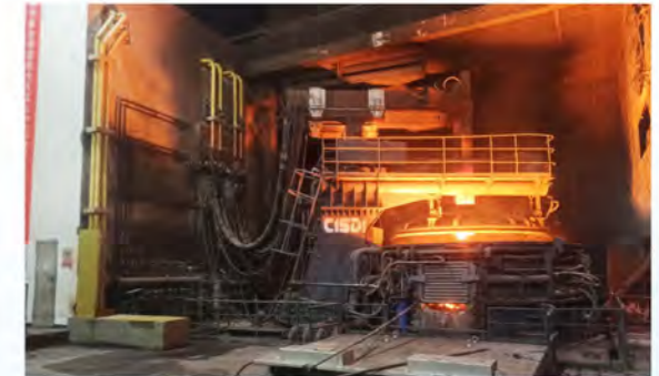
CISDI-AutoARC™, operating stably at the plant
