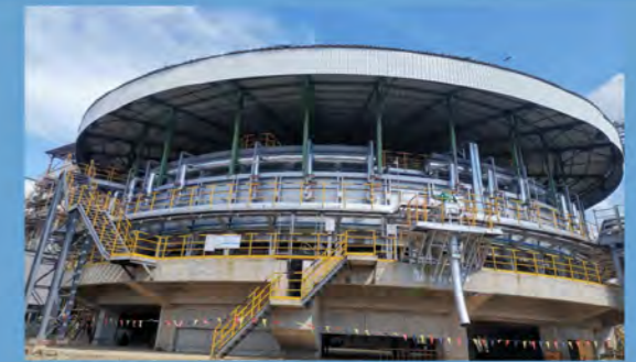
The rotary hearth furnace at Xinyu Steel in China's Jiangxi Province, which has an annual production capacity of 250,000 tonnes
